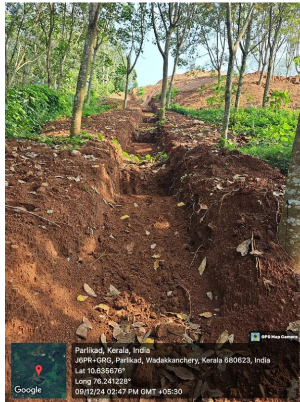
GARLAND DRAINS ALONG QUARRY BOUNDARY
