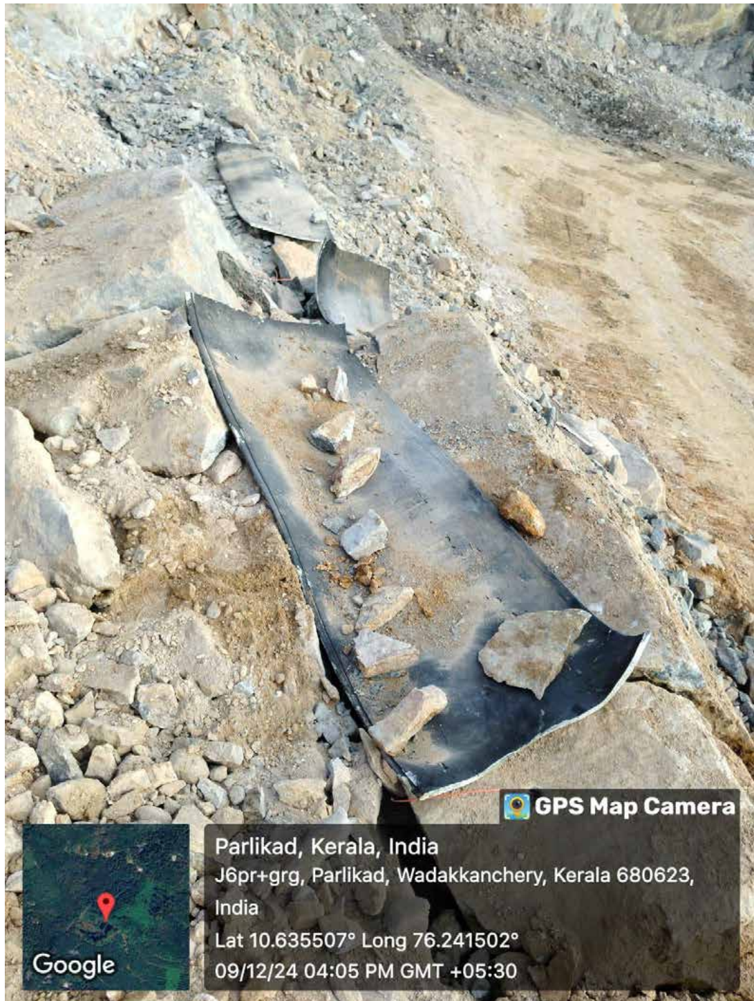
USING BLAST MATS WHILE BLASTING
